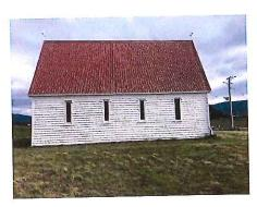
East side of the building showing the steep gable roof with modestly shaped barge boards and narrow window frames. The narrow windows forms have been coupled together to form a wider window.
