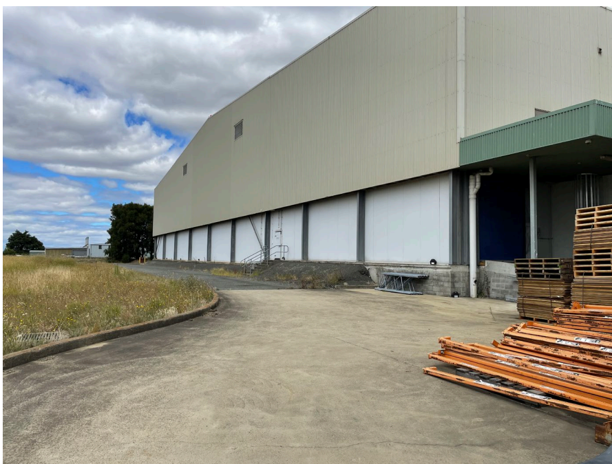
Image 8: View of rear of building
